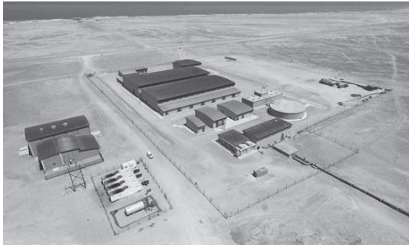
Figure 7: Erongo water desalination plant
